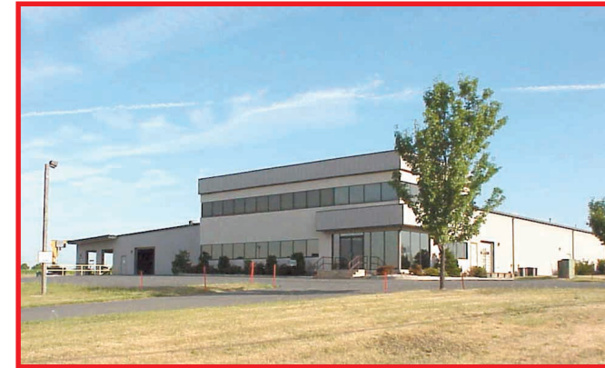
27,000 Sq. Ft. Facility
